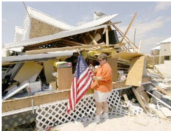
ruined house on Dauphin Island, in Mobile County, Alabama
