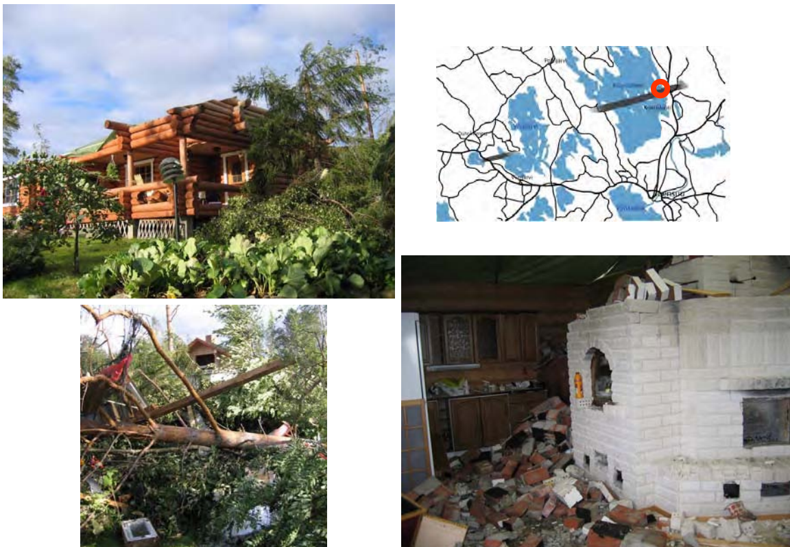
Figure 7: Damage caused by the F2 class (wind speed 50 – 69 m/s) tromb in Kontiolahti (north of Joensuu), Eastern Finland on 20 August 2004
